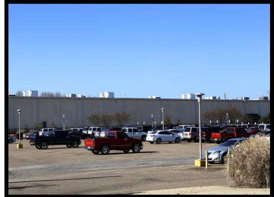
Inappropriate HVAC Screening
